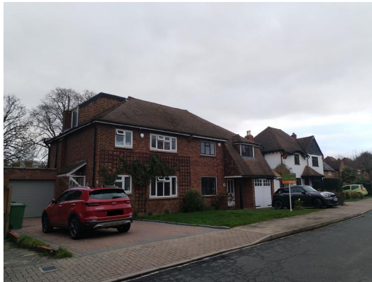
Figure 2: Photograph of host dwelling (with existing side dormer)
